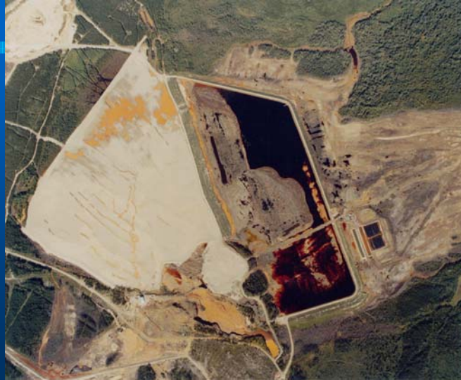
Kam Kotia Mine Site – August 2005
